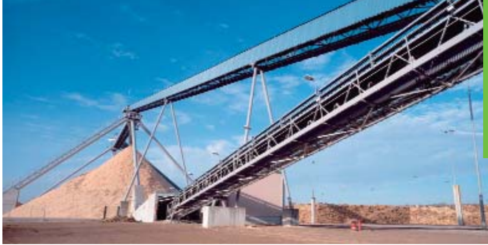
Wood is chipped before it is used for pulp production.
